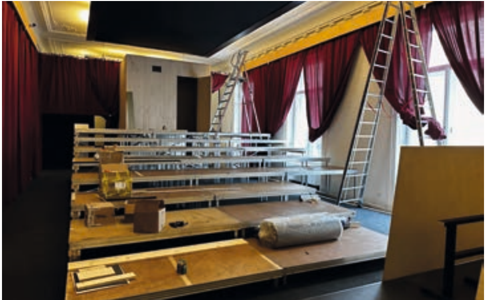
Kinosalon under construction
